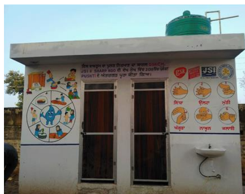
Renovated Girls toilet
